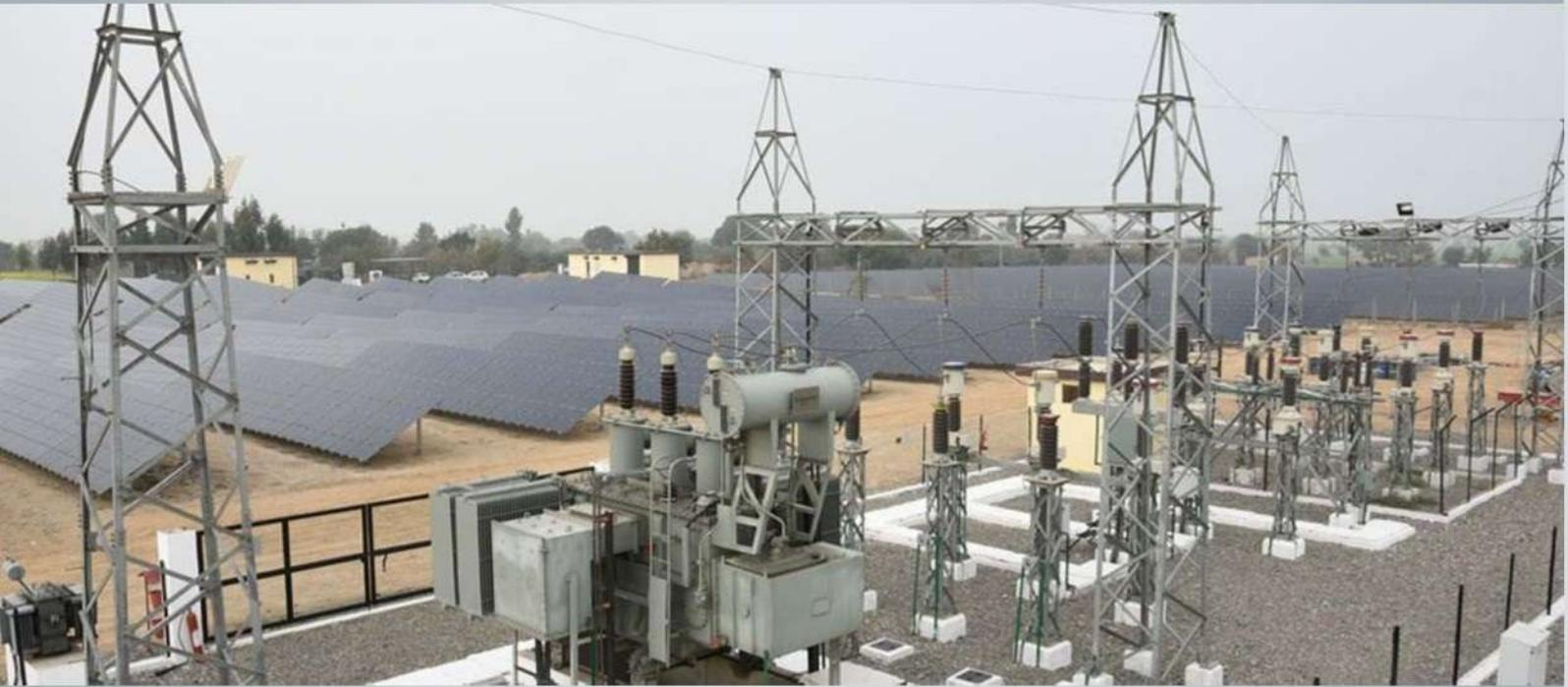
A Substation or Switchyard, is a part of an Electrical Protection & Distribution system. Substations transform voltage from high to low, or the reverse, or perform any of several other important functions.
